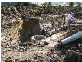
Picture of previous sanitary sewer project in Moulton.
